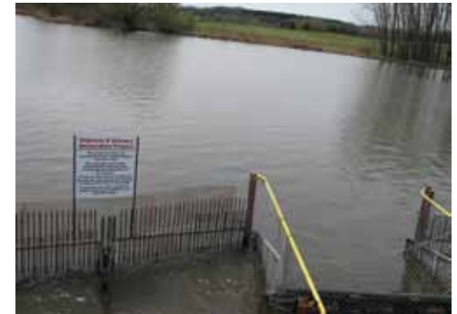
A carp barrier at the Cty. Hwy. K Bridge keeps carp from moving into the K Estuary from the lake in order to spawn.
